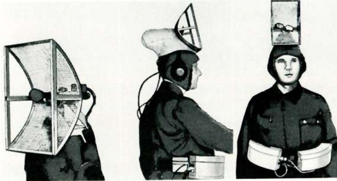
Telefunken FuMB 33 *Liliput 1* body-worn detector (2.5-3.75 GHz) for use in small craft without on-board power. The belt-worn amplifier was fragile and had poor sensitivity. Due to the 50° beamwidth, the operator “scanned” by constantly turning his head back and forth. Deployed in September 1944; 300 units built. Also issued to U-boats.
